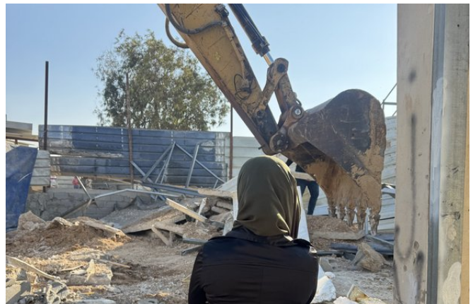
Demolished house extension
